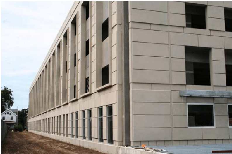
New Parking Structure for Bradley University in Peoria, IL.
