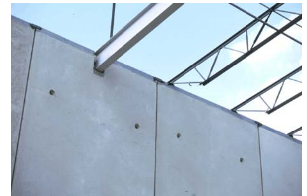
Figure 2: Loadbearing panels carry a steel roof
